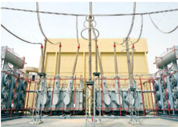
Figure 3. Converting transformer
