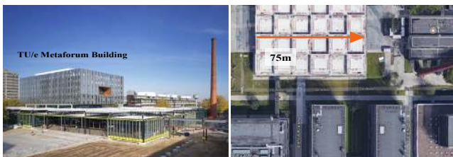
Figure 2. Fibers and antennas facilities for radio-over-fiber transmissions via the rooftop of the Metaforum building at TU/e.
