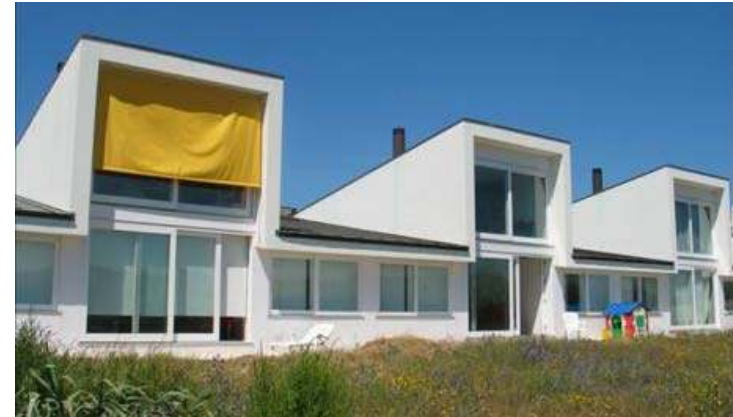
Fig. 3. 13 – Picture of existing Low Energy House in Portugal (Janas House)
