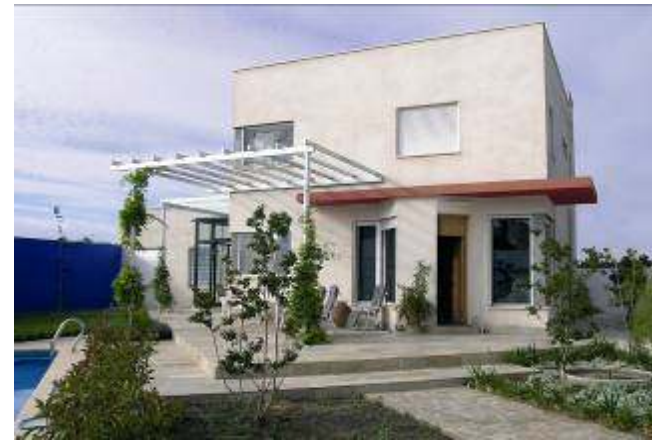
Fig. 3. 7 – Low energy housing in SP, Seville
