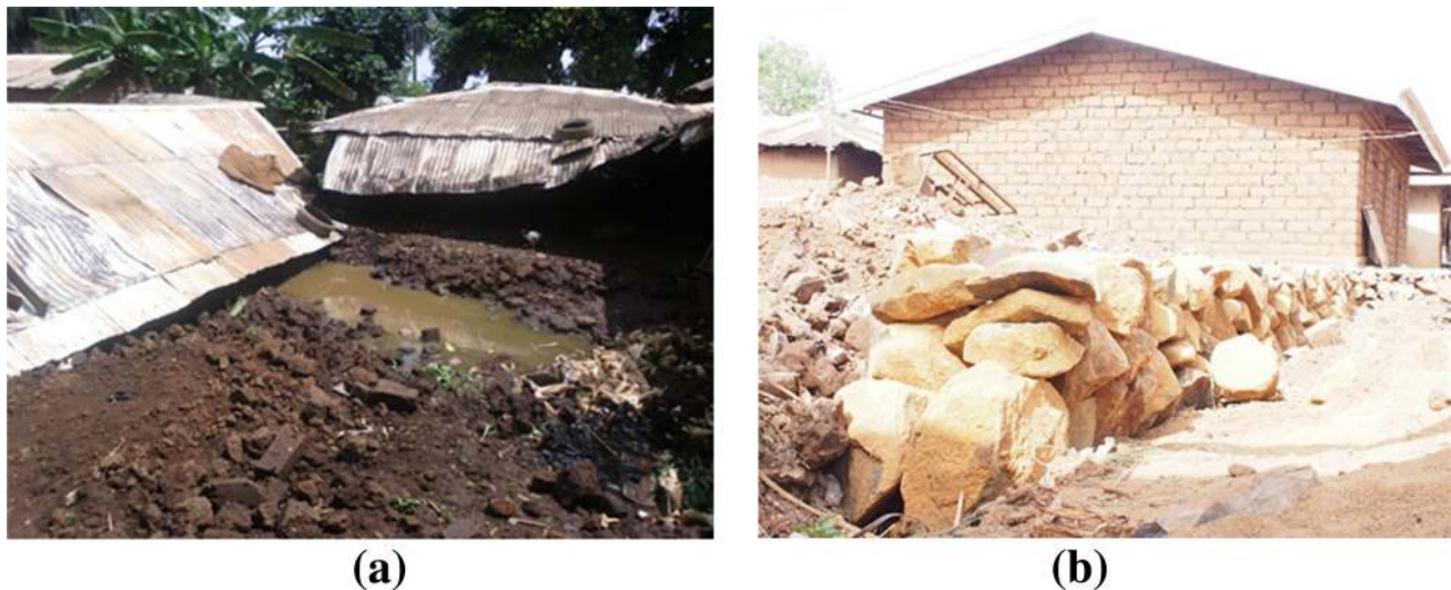
Fig. 2 Three years after the 2012 flood in Babessi—reconstruction of destroyed mud-brick houses still ongoing. a Destroyed mud-brick houses after the flood in 2012; b Reconstruction of houses with stone-
