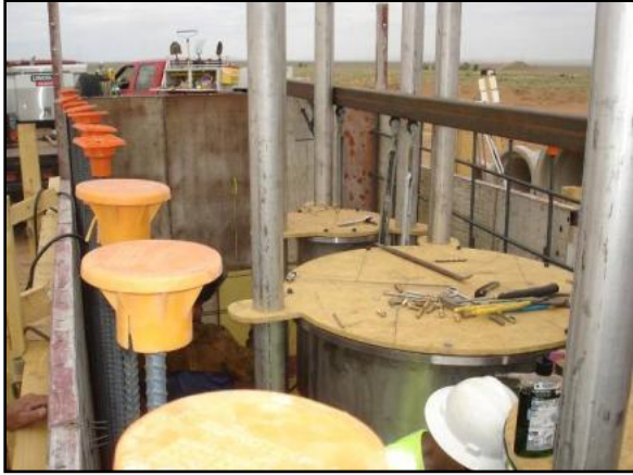
forming the thrust block around SS elbows
