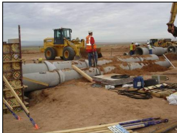
laying the three rows of RCP
