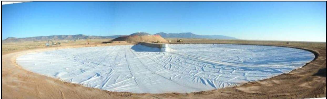
Figure 39 Installation of the water pool liner.
