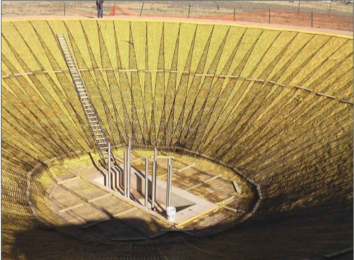
Figure 28 Cavity with polyurethane foam and carbon reinforcement mesh liner.
