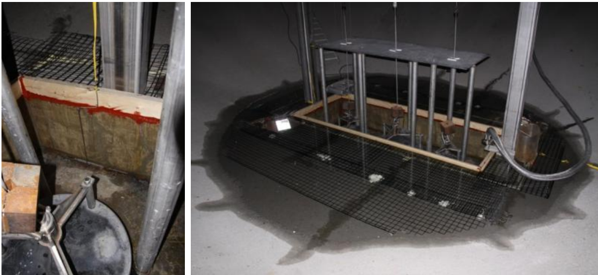
Figure 166 Construction and installation of the ice shield on the reservoir floor.
