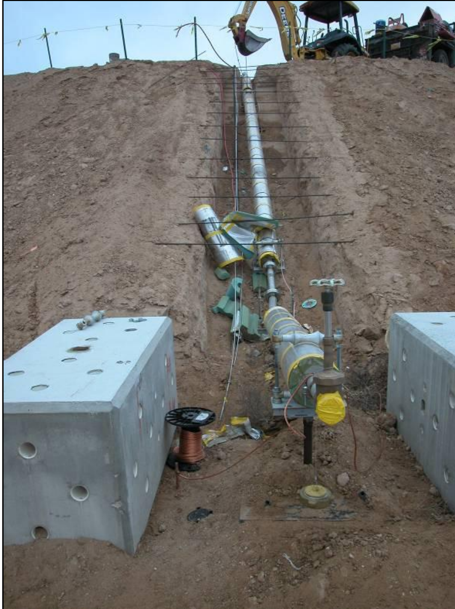
Figure 40 LNG fill pipeline in construction.
