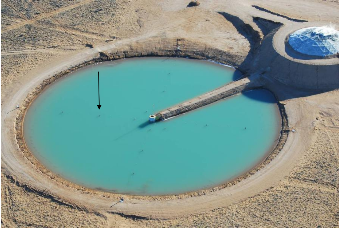
Figure 51 DFTs in pool the morning of Test 1.
