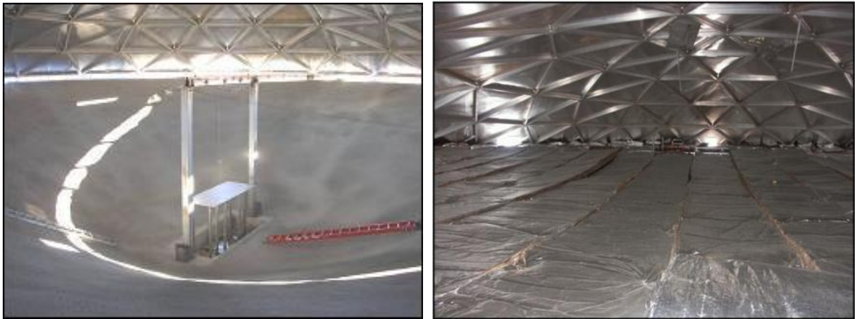
Figure 160 Reservoir without ceiling and reservoir with ceiling.
