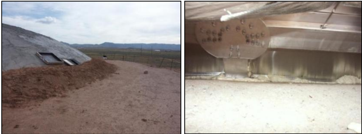
Figure 161 Minimizing air leakage at dome/reservoir interface and at flashing gaps.
