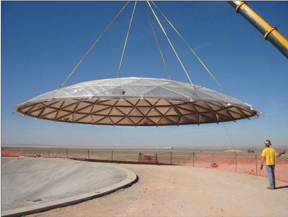
Figure 30 Installing the aluminum dome (with wire mesh) on the reservoir.
