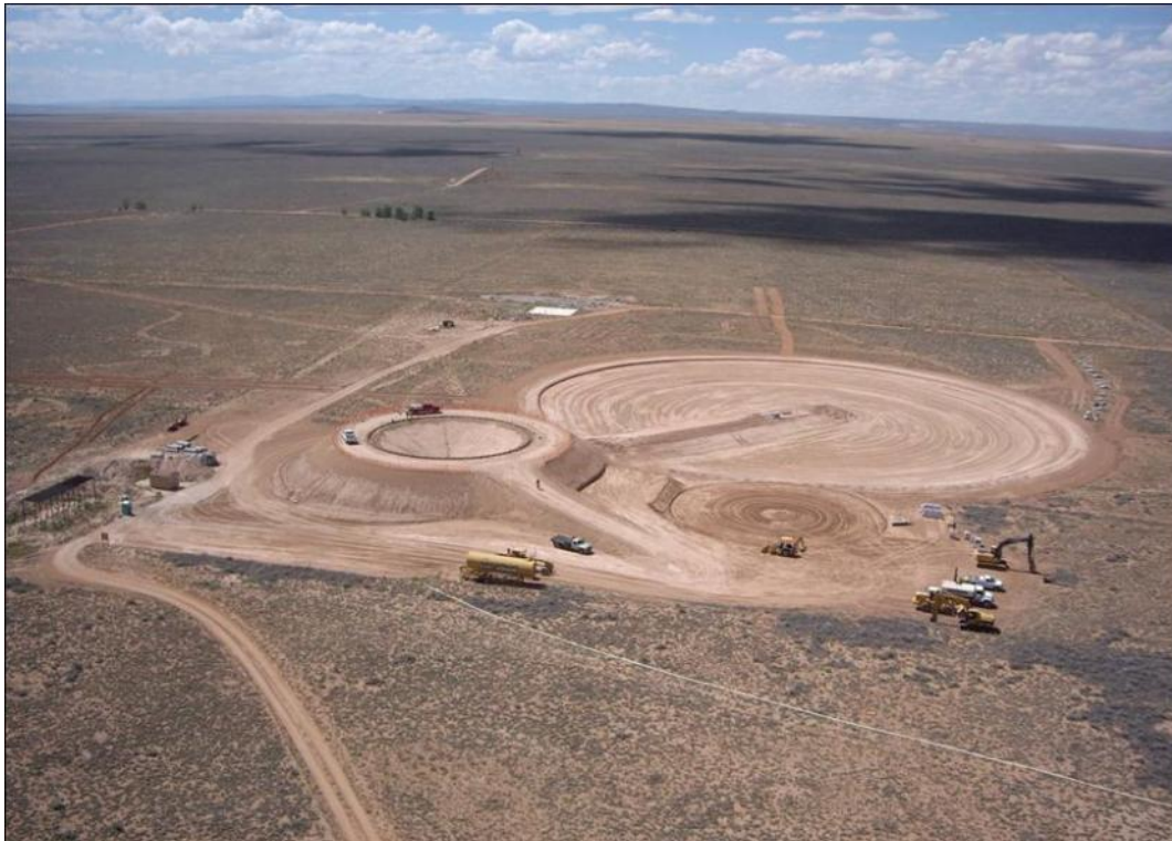
Figure 26 Water pool excavation and reservoir construction.
