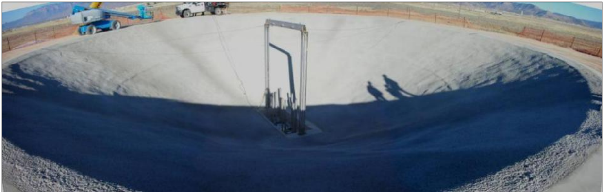
Figure 29 Completed reservoir cavity with shotcrete liner.
