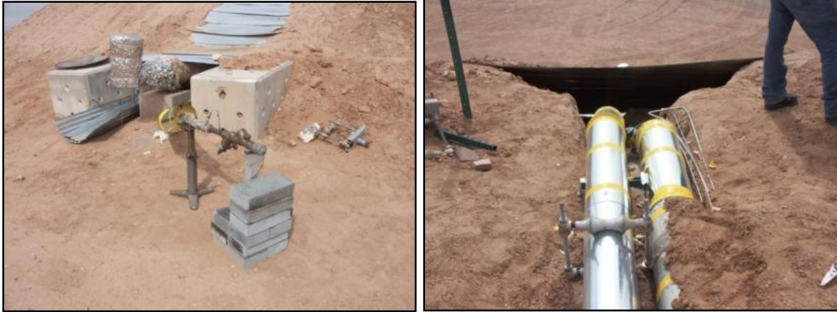
Figure 163 Building the LN 2 spray line coupler and pipe external to reservoir.
