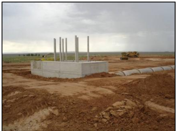
completed thrust block at base of reservoir
