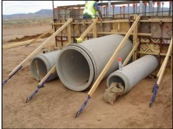
1 st set of reinforced concrete pipe (RCP)
