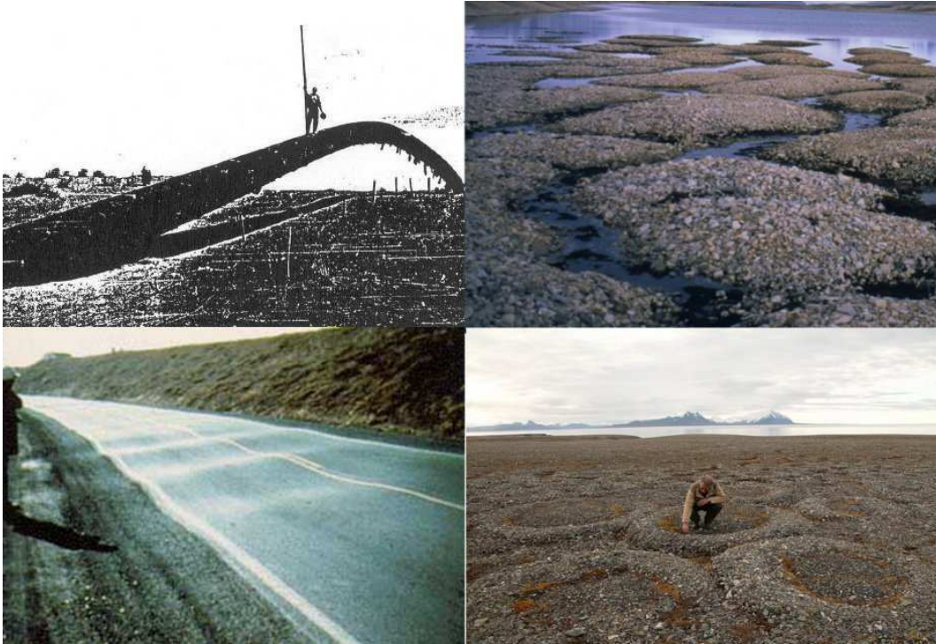
Figure 1: Phenomena caused by frost heave. Clockwise from top left: a pipeline heaved out of the ground [3], hummocks, stone circles and road buckling [2].
