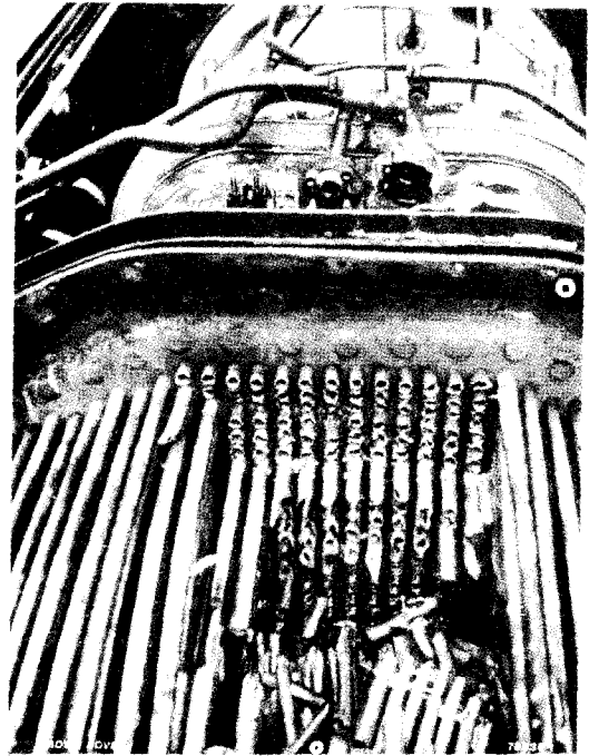
Fig.13 Fire damage in gas turbine locomotive tubular recuperator (by courtesy Brown Boveri) (68-4742)
