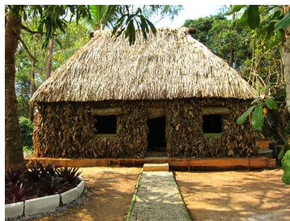
Note) Photo was taken after the completion of the Fijian traditional construction at CATD, Fiji on September 2011 by the author
