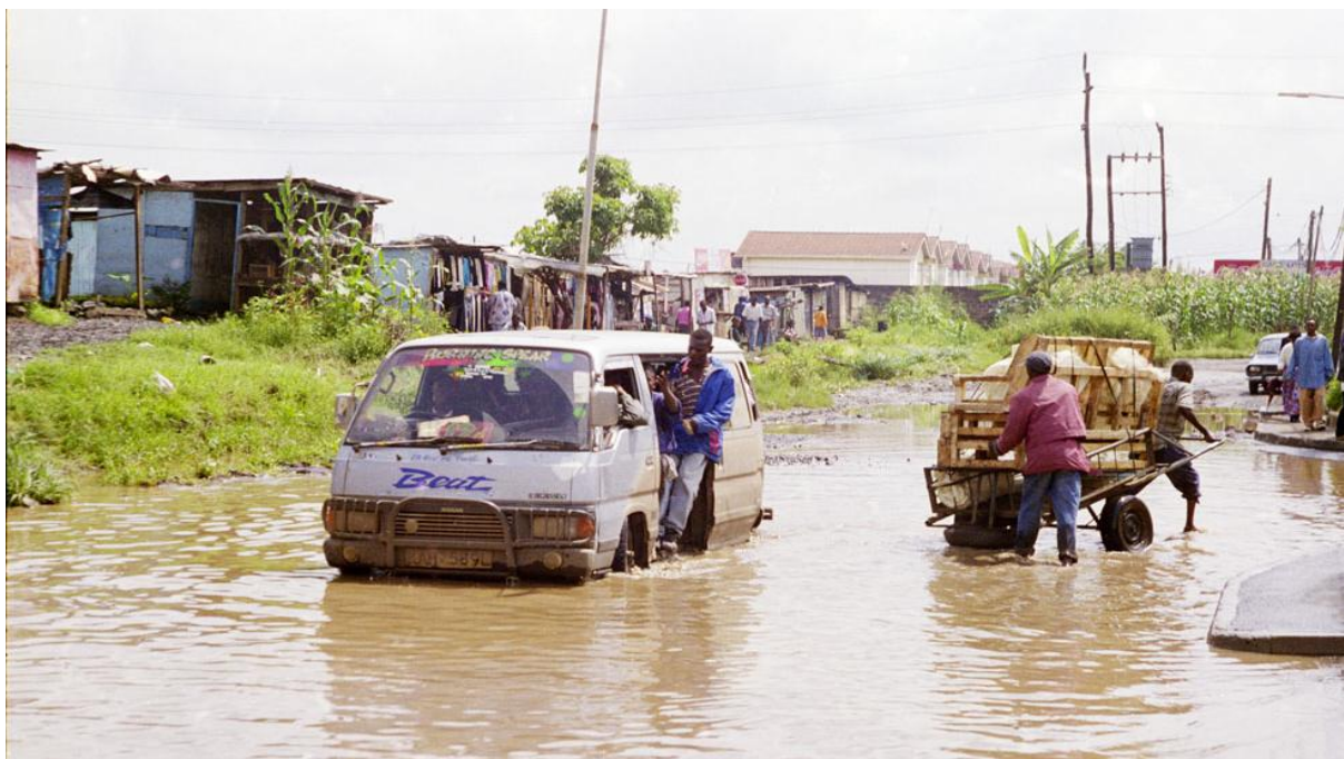
Figure 4.2: A section of a desperately in need of maintenance road in Nairobi's Eastlands in the 1990s (photo Courtesy of Antony Kaminju).
