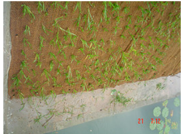
Fig. 8. CGG, third day of installation.
