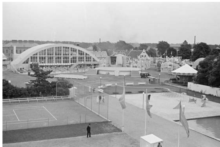
Fig. 2 View of the exhibition area, with a tennis court in front and the arched building containing the main restaurant in the background. Fritiden , July 15/16 1936. Photo: Gunnar Lundh (GL.113332).
