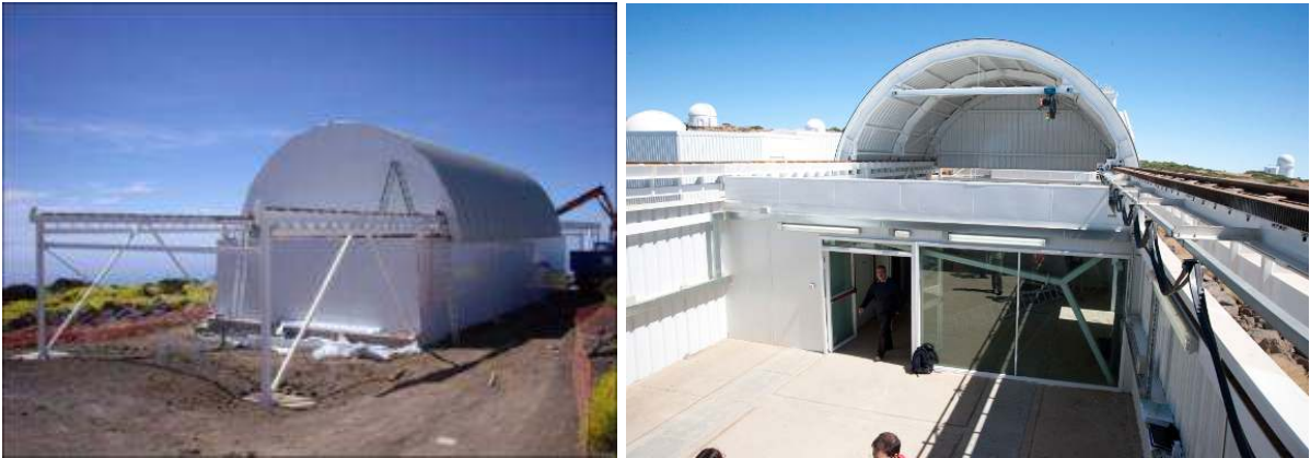
Figure 2. Left: QUIJOTE-CMB enclosure at the Teide Observatory. Right: Inside the QUIJOTE-CMB dome, before the installation of QT1.
