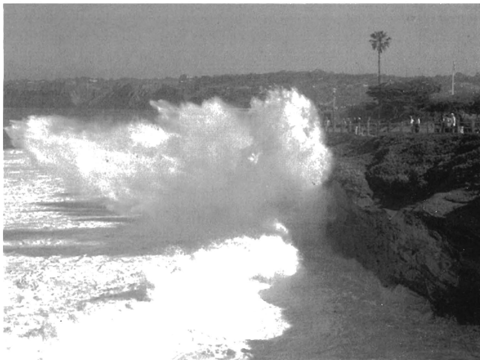
Figure 10. The La Jolla site on January 30, 1998 showing wave hammering of the cliff face at high tide. These cliffs have remained essentially stable over much of this century despite being frequently attacked by large waves that break relatively close to the cliffs.
