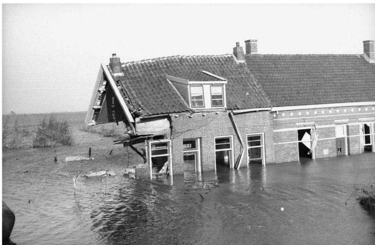
Figure 3. Image of heavily damaged house during 1953 North Sea flood in Zeeland, the Netherlands. Source: Commons Wikimedia.
