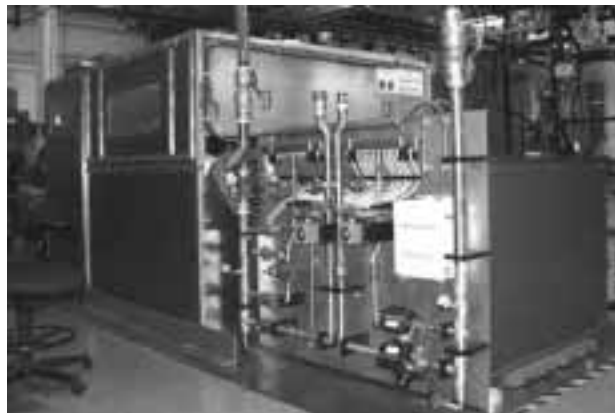
Figure 5: The prototype 140 kV power supply has been tested to full peak power.
