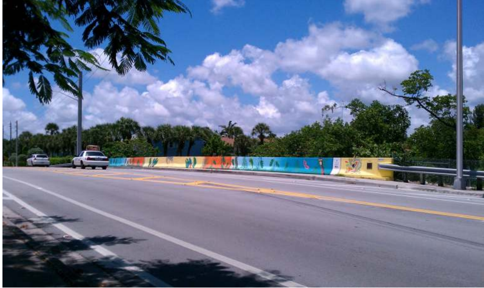
Figure 46. Bridge adjacent to Colohatchee Park on N.E. 15th Ave. looking south. Photo by Emma Ergon 2011
