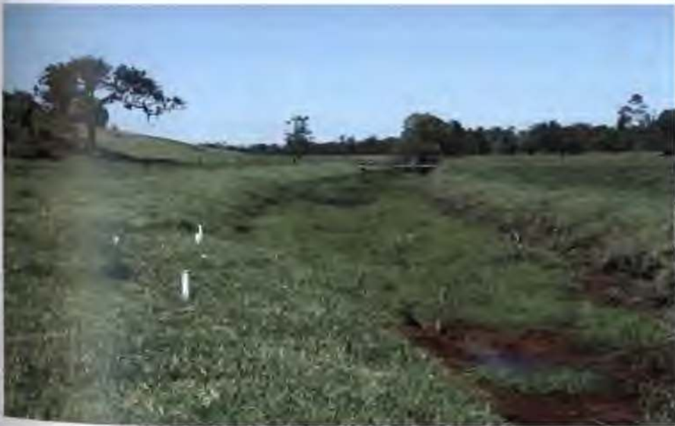
Plate 4.2: Flood mitigation drain at the lime-fly ash barrier study site looking downstream. Drain width is approximately 5m
