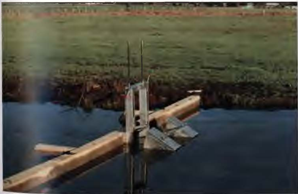
Plate 2.2: Self-Regulating Tilting Weir (built in 200 by UOW Acid Sulphate Soils Research Team)
