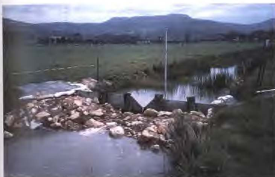
Plate 2.1: High v-notch weir
