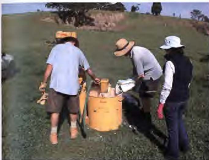
Plate 5.7: Mixing of lime-fly ash/water slurry.
