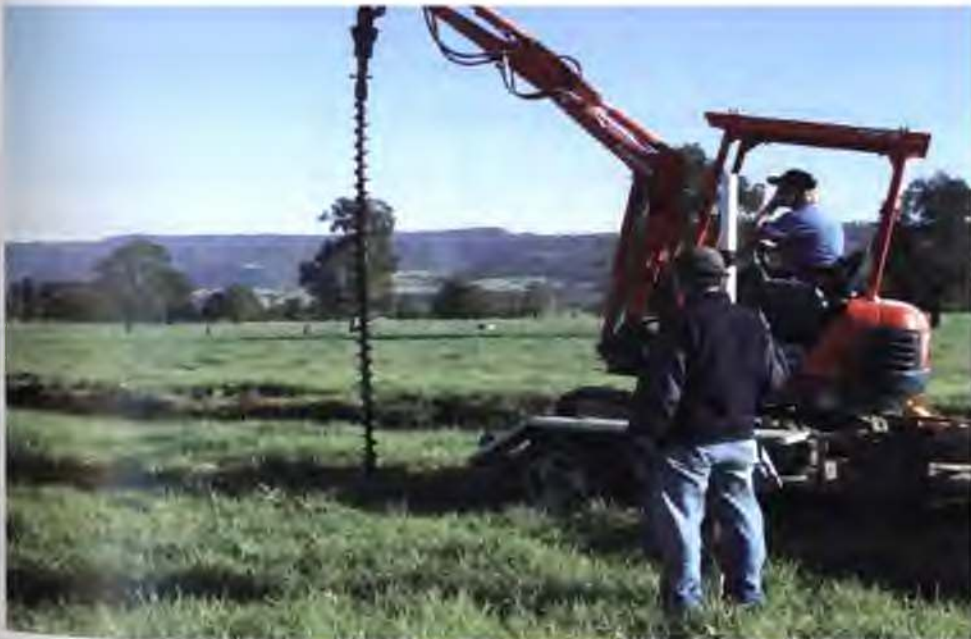
Plate 4.8: Drilling of Piezometer Holes
