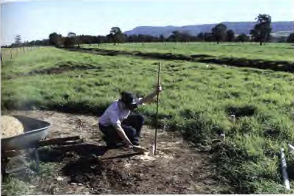
Plate 4.6: Installation of Observation Holes by the author.
