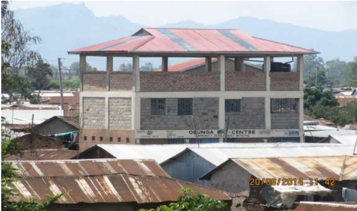
Figure 6.3 Obunga Water Scheme Office (Source: Author)
