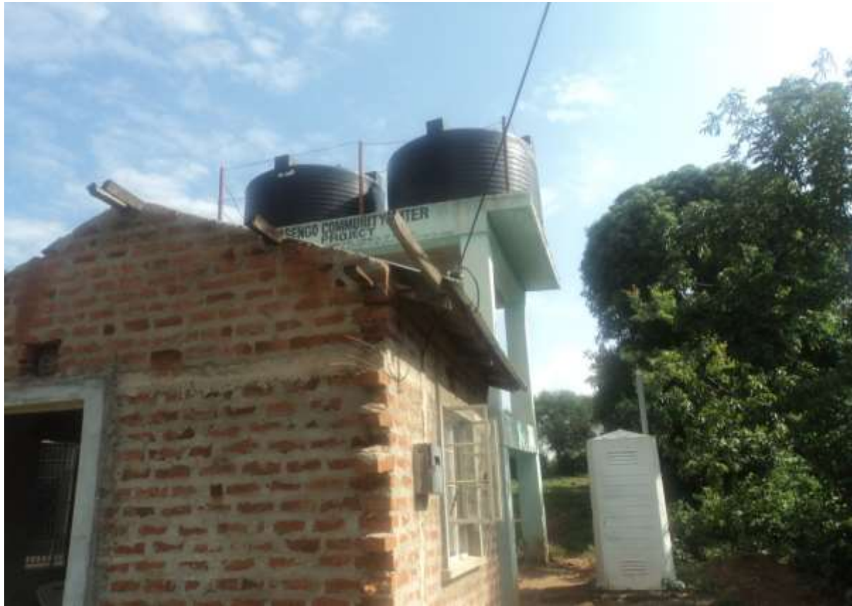
Figure 6.1 Asengo Water Scheme Office (Source: Author)
