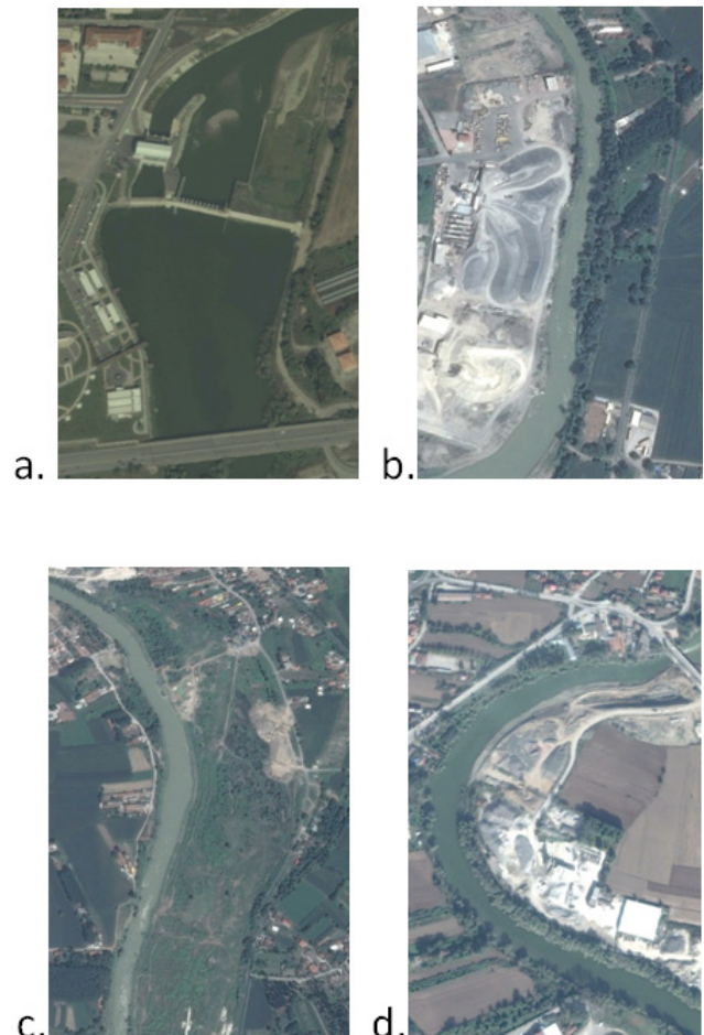
Figure 4. Photograph shows anthropogenic impacts of the study area, (a) Sakarya HES Dam; (b) Instream sand mining operation; (c) Unserviceable instream mining operation; (d) The Historic Sakarya Bridge crossing Sakarya River
