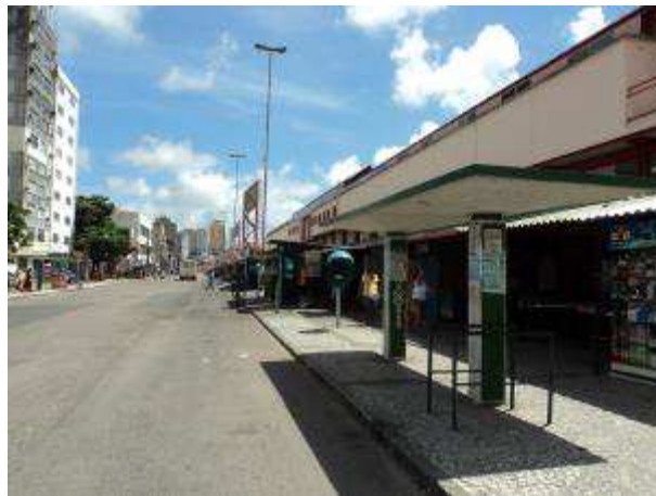
Figure 34: Precast concrete shelter
