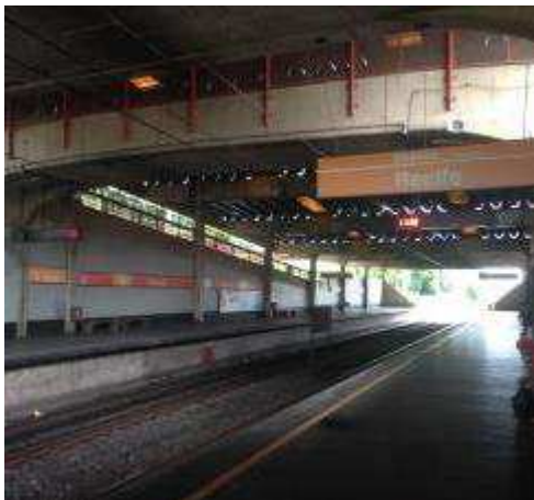
Figure 38: Metro station: inside view
