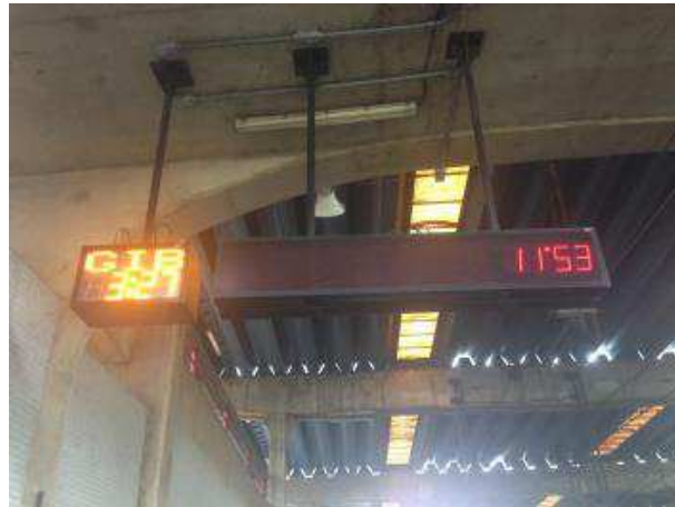
Figure 42: Metro station: real time information
