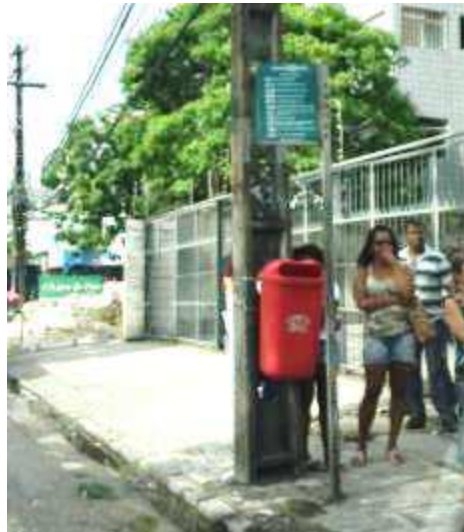
Figure 32: “L” columns bus stop
