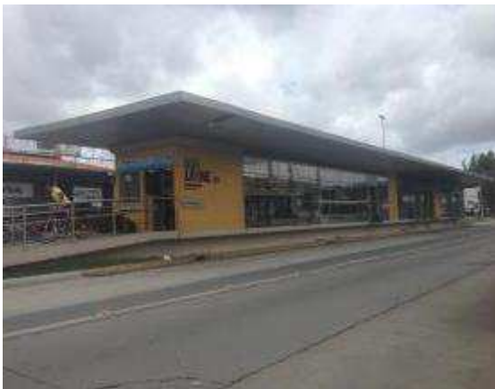
Figure 35: BRT station: overview
