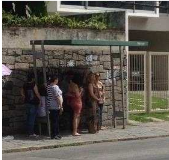
Figure 33: Metal shelters bus stop
