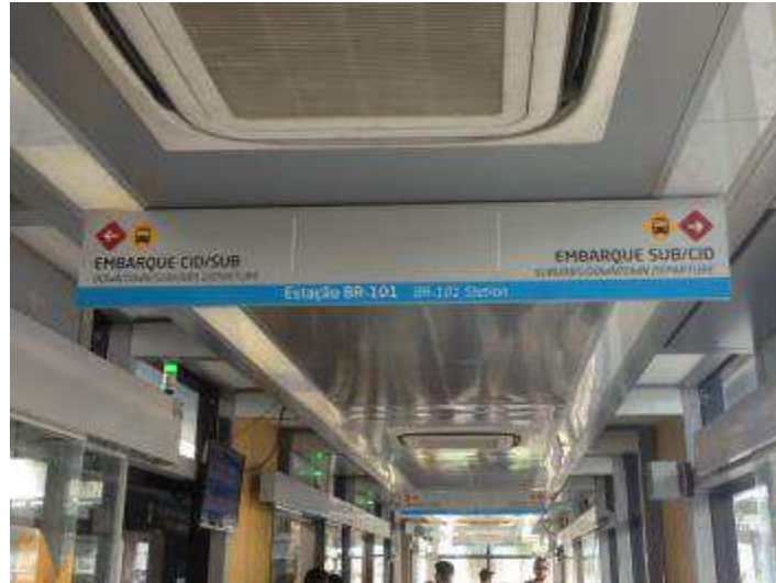
Figure 37: BRT station: inside view
