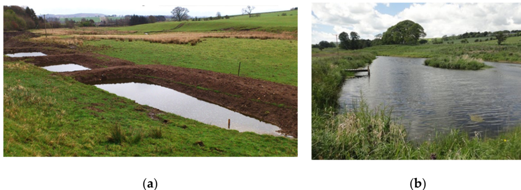
Figure 8. (a) In Netherton Burn (Northumberland), a ditch has been modified to create sediment traps [51] and (b) a permanent pond with 1m of available flood storage. This RAF protects a larger flood storage pond immediately downstream which provided the main RAF storage requirements.
