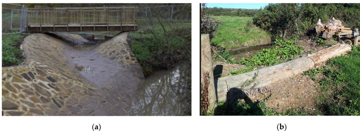
Figure 5. Draw off structures at Coatham Woods lowering the bank, Co. Durham (a) and SloWaters Project Co. Wexford, Ireland (b) raising the overflow level [48].
