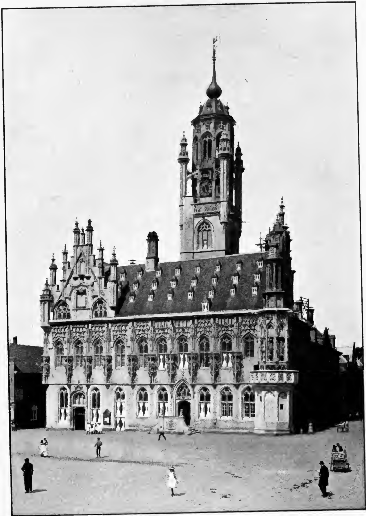
THE MARKET PLACE AT MIDDELBURG.
