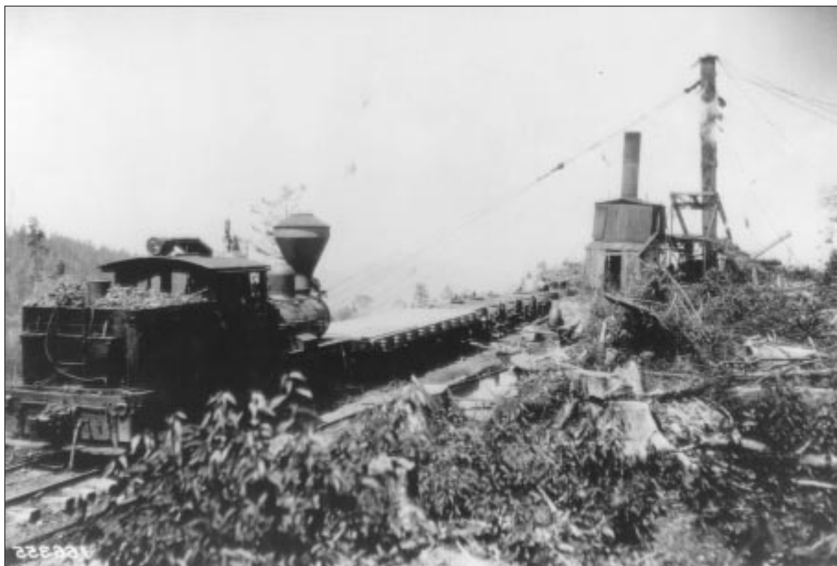
Figure 12—Lidgerwood high lead skidder and Shay locomotive used for logging in the Pigeon River watershed in western North Carolina. (USDA Forest Service photograph.)
