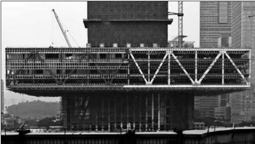
Figure 10.9. Exterior of Shenzhen Stock Exchange. Video still from Zachary Formwalt, Unsupported Transit , 2011.
