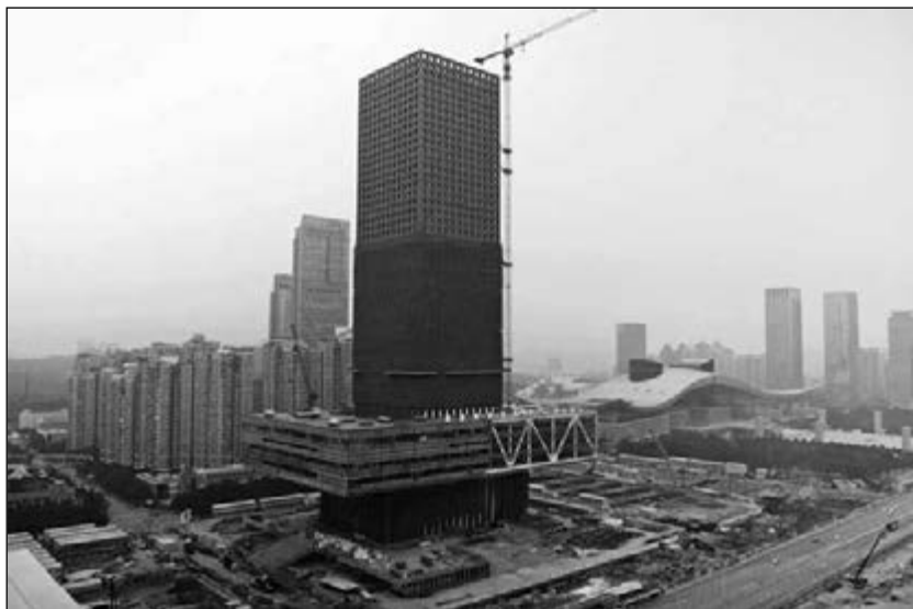
Figure 10.4. Exterior view of the Shenzhen Stock Exchange in China under construction. Production still from Zachary Formwalt, In Light of the Arc , 2013.
