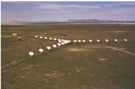
Figure 1: The VLA antennas in one of its array configurations. The antennas can be transported to provide either more compact or more spread-out configurations. (Image from NRAO / AUI / NSF).
