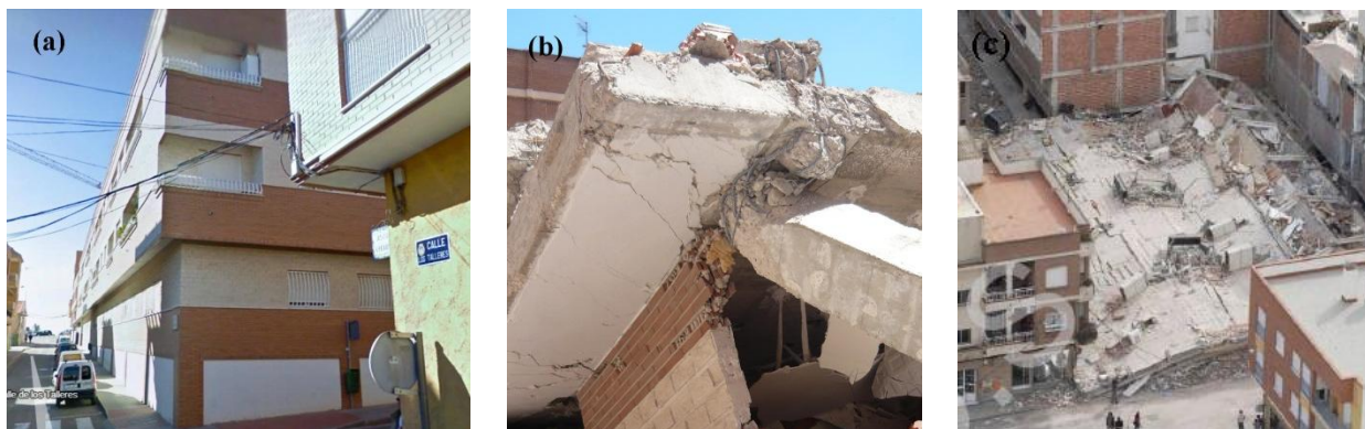
Figure 10. The only building collapsed due to the Lorca earthquake, before (Google Street View) (a) and after the event (b), (c). Photograph (c) adapted from Regalado (2011).
