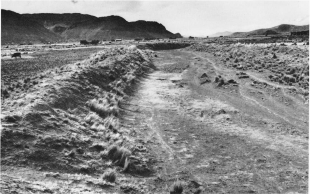
Figure 5. Artificial earthen levees designed to stabilize extracted river flow on the Río Catari canal by-pass (see Figure 4, Feature 2). These reinforced earthen banks are also characteristic of the Waña Jawira River shunt in the valley of Tiwanaku.
