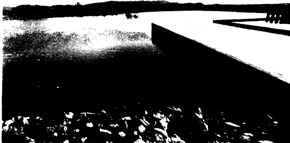
Figure A6. Effluent holding pond with chlorine contact tanks at right. The high-quality effluent permits split-stream treatment during wet weather. The TF/SC effluent is mixed with primary effluent in the holding basin. The mixture meets ocean discharge requirements for wet weather and is discharged with the outgoing tide through a submarine outfall. (Source: Brown and Caldwell Consulting Engineers. Used with permission.)
