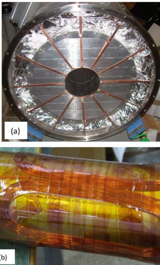
Fig. 6. (a) Cryogenic intervention at the TwinEBIS magnet with the iron shield dismantled (two bars at the bottom remaining) and the cryostat partly open. The photo shows the addition of radial copper strips that effectively connects the liquid nitrogen jacket to the 80 K tube, which shields the liquid helium jacket from the room temperature bore tube. (b) Photo of the transverse steering coils located between the cooling mantle and the solenoid bore as of 2016.
