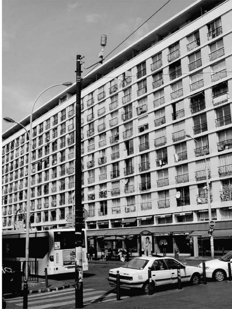
Figure 11. Example of a shielded T-RH sensor assembly at a site in the city centre.
