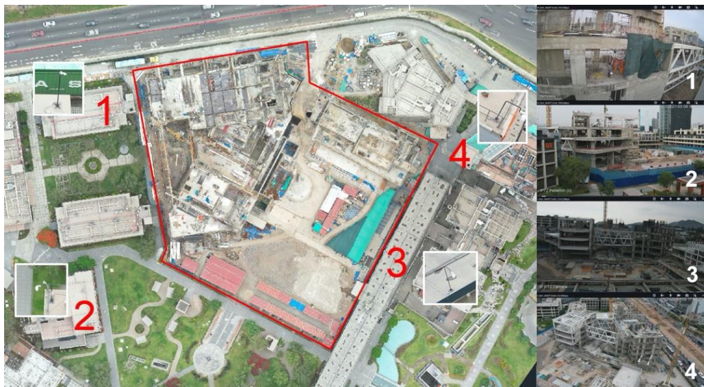
Figure 1. General plan of the construction site showing the location of the four cameras (left), and an example of the images obtained from each camera (right)
