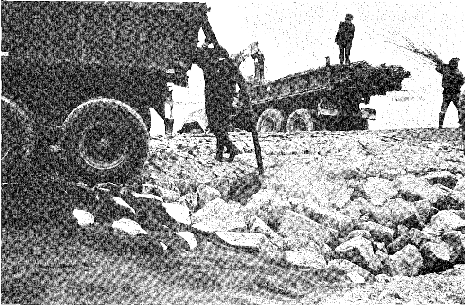
Photo 16 Grouting a crushed stone layer directly from an asphalt container truck
