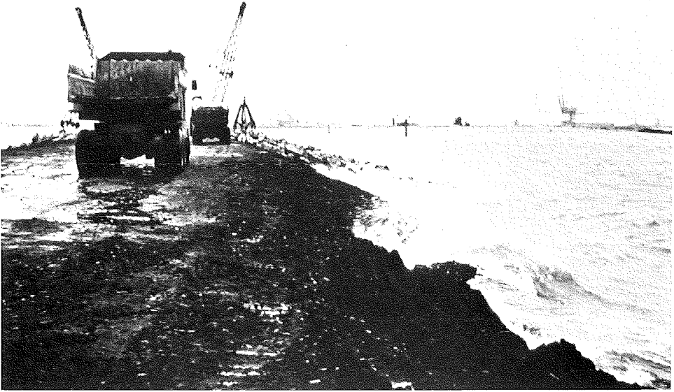
Photos 25, 26 Construction of a lean sand asphalt reclamation bund
