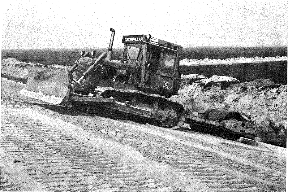
Photo 4 Compacting the sandbed using a vibratory roller
