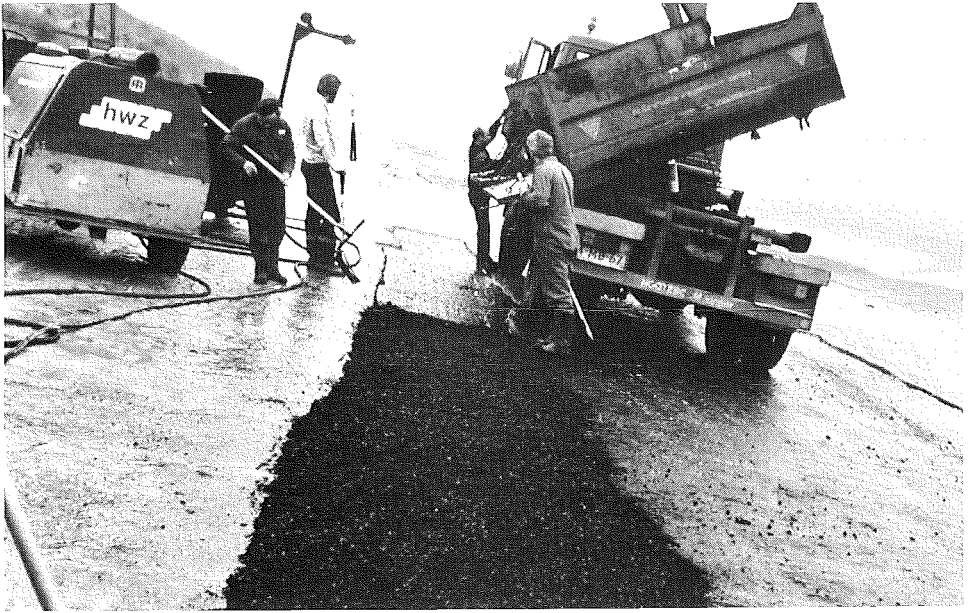
Photo 31 Repairing the seriously damaged surface of an asphaltic concrete revetment: The fraised area is refilled with asphaltic concrete
