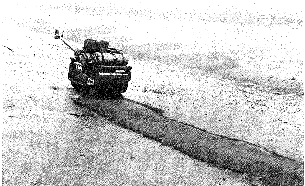
Photo 32 Repairing the seriously damaged surface of an asphaltic concrete revetment: The refilled area is compacted with a tandem vibratory roller
