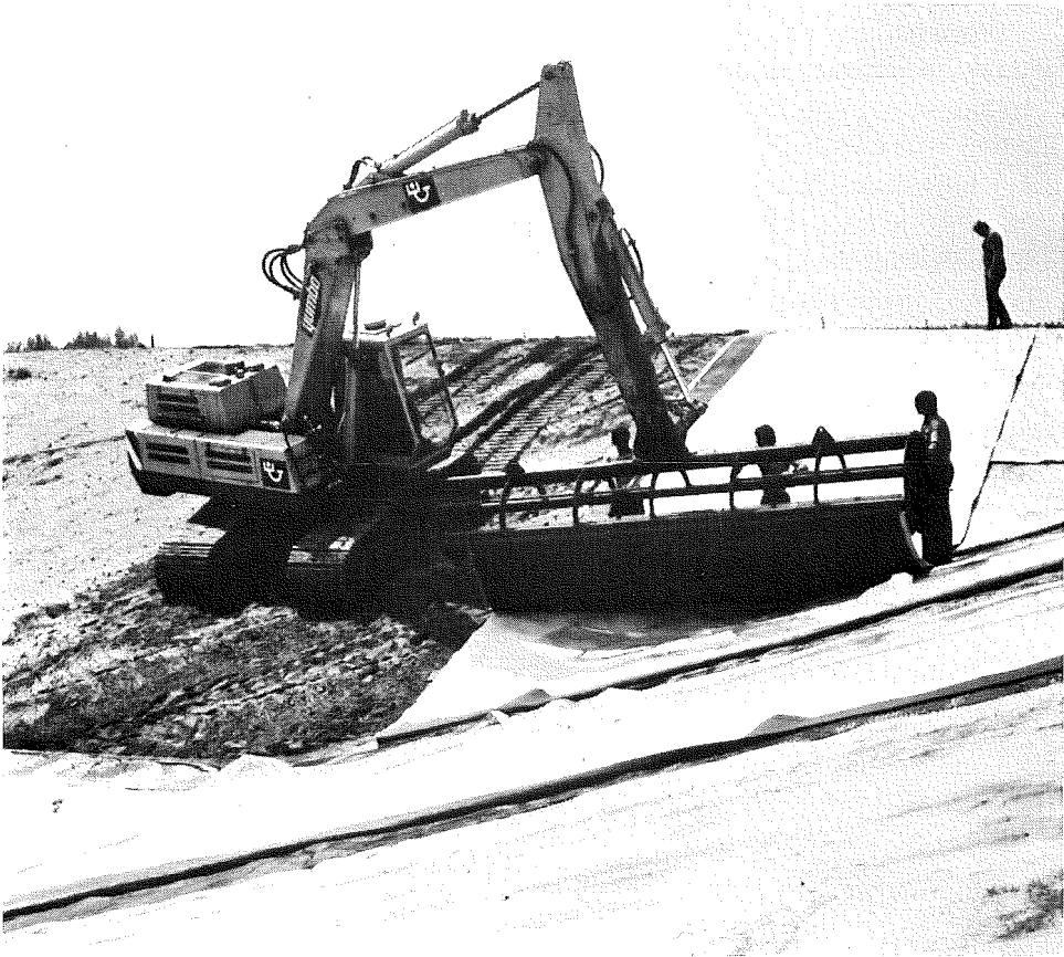
Photo 28 Placing a prefabricated membrane (Hypofors)
