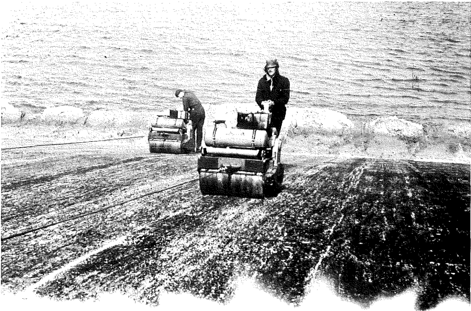
Photo 14 An asphaltic concrete revetment being compacted with a tandem vibratory roller
