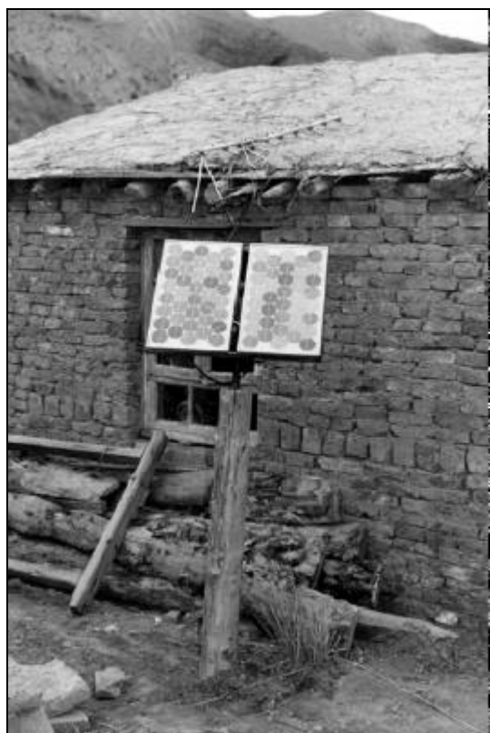
Figure 1. Solar home system installation in Xinjiang Province, typical of such installations in China.
