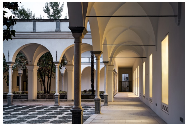
Figure 3. Picture of the Patio at the ground floor
