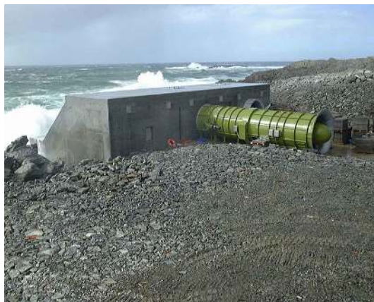
Figure 3. LIMPET, a shoreline OWC, developed by Wavegen [9]. In operation since 2000.
