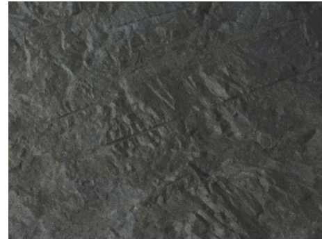
FIGURE 15: Optimized smooth blasting effect of Grade III surrounding rock.
