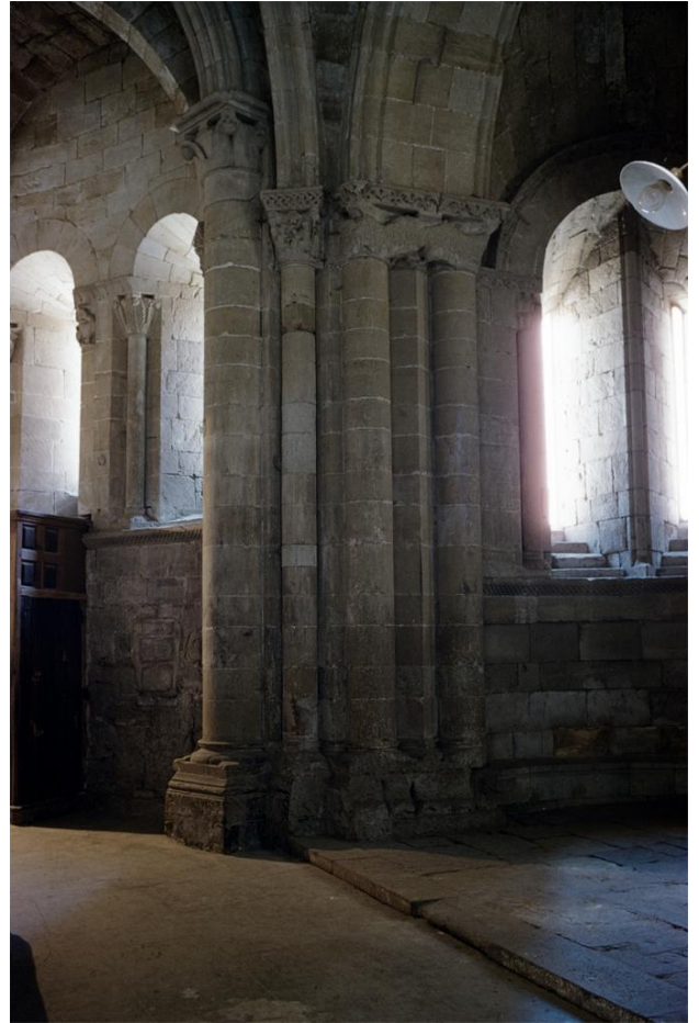
Figure 4.17: Compound piers at Canterbury Cathedral, England (left), and Cathedral of Santo Domingo, Calzada, Spain (right).
