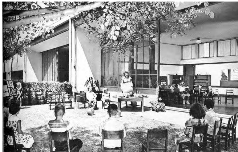
Corona Avenue School, Bell, California, 1935 by Richard Neutra incorporated the first application in the United States of a sliding glass door, essentially combining indoor and outdoor classroom space. 23
