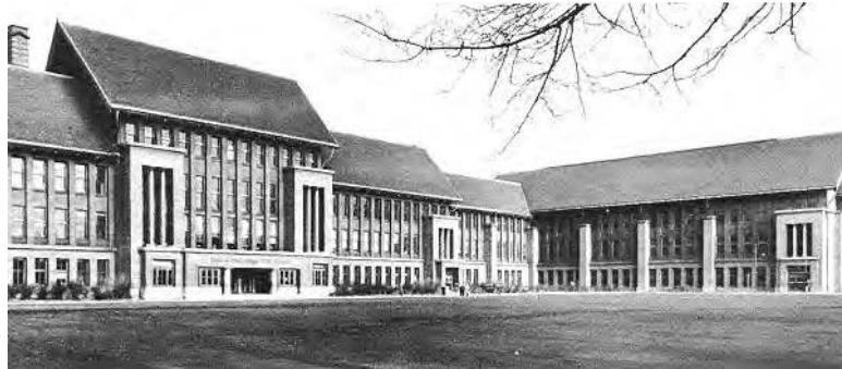
Carl Schurz High School, Chicago, 1910 by Dwight Perkins displayed no ornament or historical eclecticism and is perhaps the earliest example of open-planning in schools where parts of the same school are differentiated to house various activities. 22
