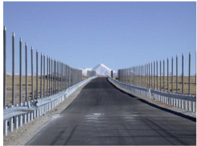
Figure 5. Permafrost preservation—in this case to stop subsidence of a road—will increase in importance as global warming affects the permafrost ‘table’. Reprinted from Zhang et al. [3] with permission from Elsevier.
