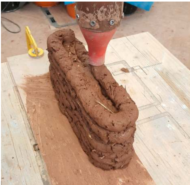
Figure 4. The Layer by layer technique of printing.
