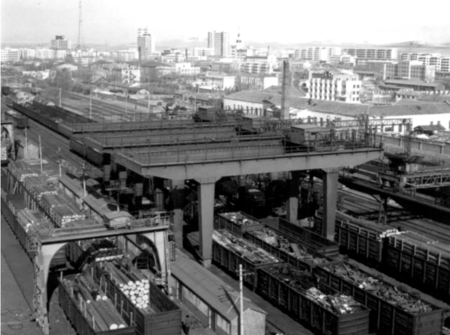
Large gantry crane in busy freight reloading yard at Manzhouli Station on Russian border (China's Railways Press)
