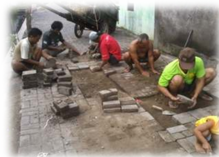
Fig. 5: Community participation in the repair of roads damaged by floods
