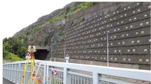
Fig. 3 Laser scanning location
