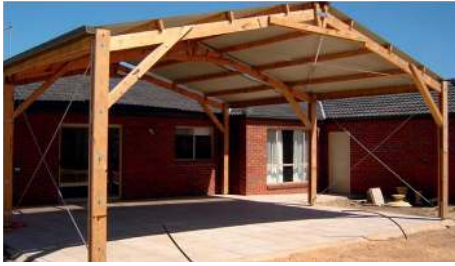
FIGURE 1: Typical timber portal frames.
