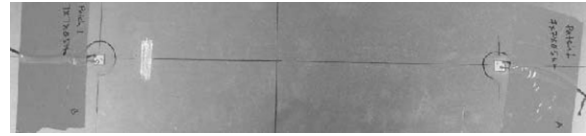
Figure 15. Surface damage at 32 mm from the actuator.
