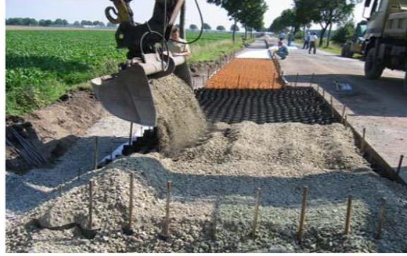
Figure 2. 14 Installation and infill of the geocell (Kief et al. 2008)
