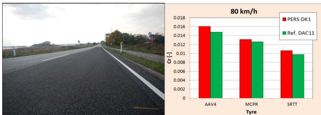
Figure 12. Danish test section with PERS-DK1 surface together with the obtained values of the rolling resistance coefficient on PERS and on the reference DAC11 at the speed of 80 km/h [3]
