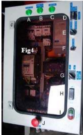
Figure 6-5 Components of control panel.
