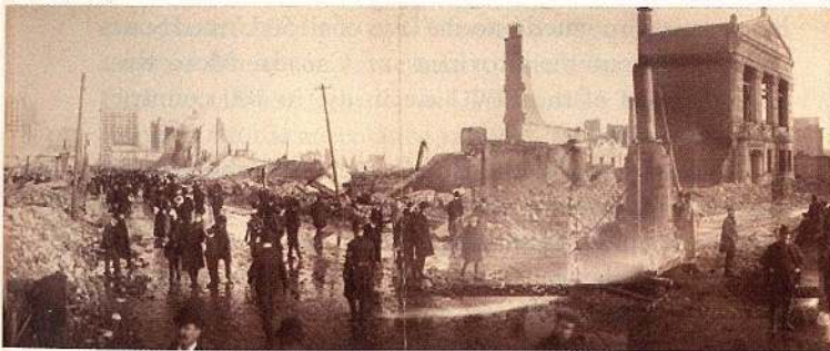
▲ Because their hose fittings were incompatible, many firefighters could only stand and watch Baltimore burn in 1904.
