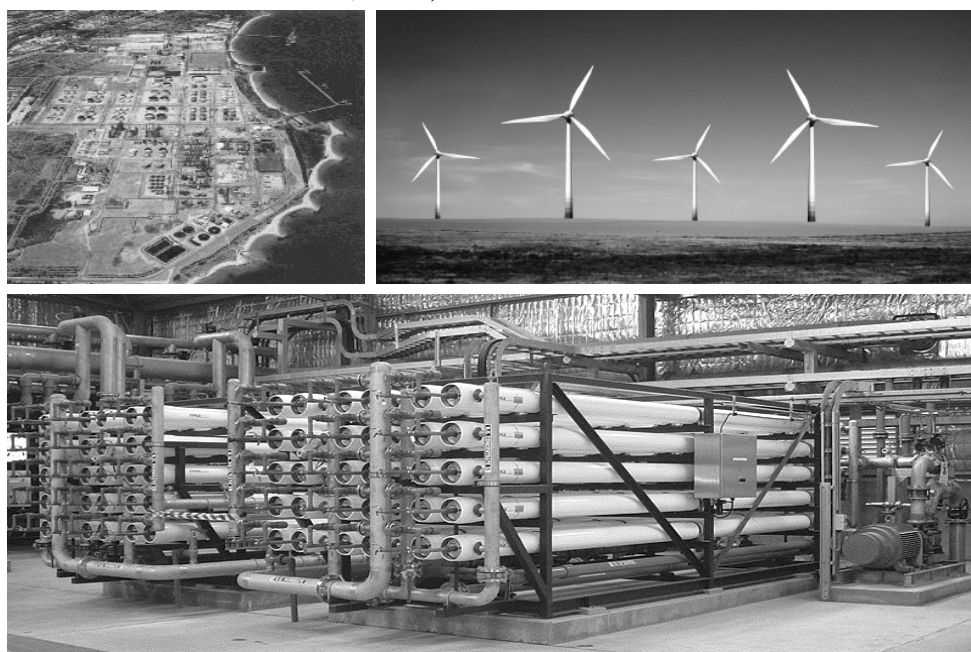
Figure 3. The Kwinana Seawater Reverse Osmosis Desalination (SWRO) Plant and Wind Farm in Perth, Western Australia. 3a ( Upper Left ) The SWRO Plant seaside location in Perth; 3b ( Upper Right ) The Emu Downs Wind Farm consisting of 48 Vestas wind turbines each with 1.65 MW generating capacity; 3c ( Lower ) The desalination plant, with 12 SWRO trains with a capacity of 160 megalitres per day and six BWRO trains delivering a final product of 144 megalitres per day. (Pankratz, 2008).
