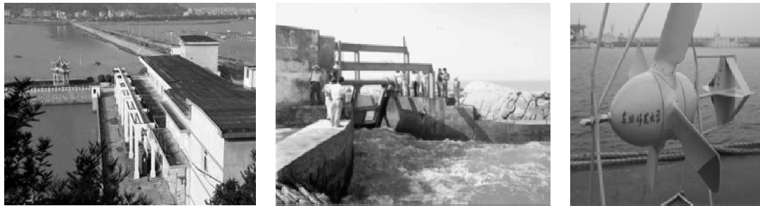
Figure 4.. LHS : Jiangxia pilot tidal plant (Photo by Zhou Xuejun). Middle : The pendulum-type wave energy conversion device in Dagan Island (100 kW, 2000, NOTC). RHS : 2 kW device for surface tidal current (2009, NENU) (Wang et al., 2011)
